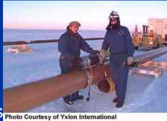
Photo Courtesy of Yxlon International
